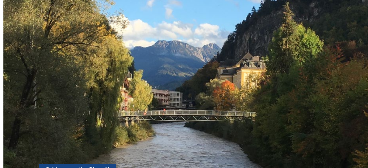
Bridge over the River Ill
